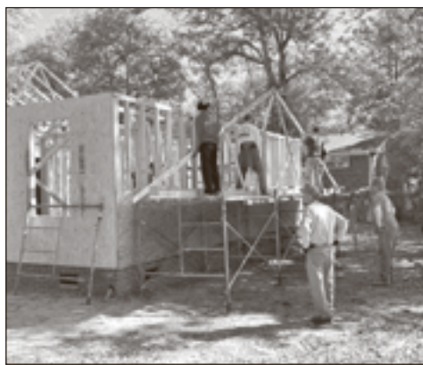
TRUMC did five days of the onsite work.
